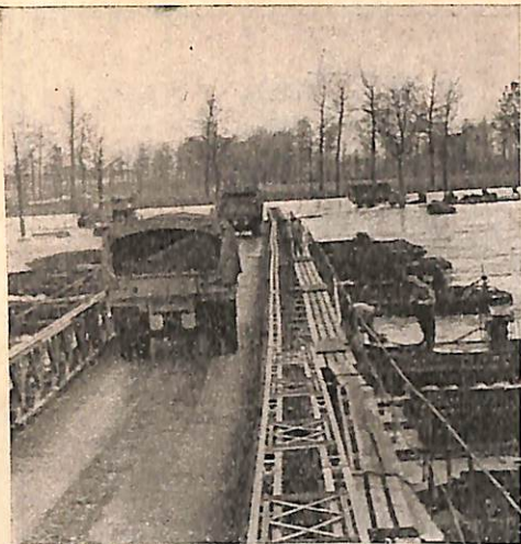
CROSSING THE RHINE. When Allied forces crossed Hitler's great Rhine water barrier with "ease" the fate of Germany was spelled out in capital letters. Trucks of 3414 are shown crossing on a Ponton Bailey Bridge.
